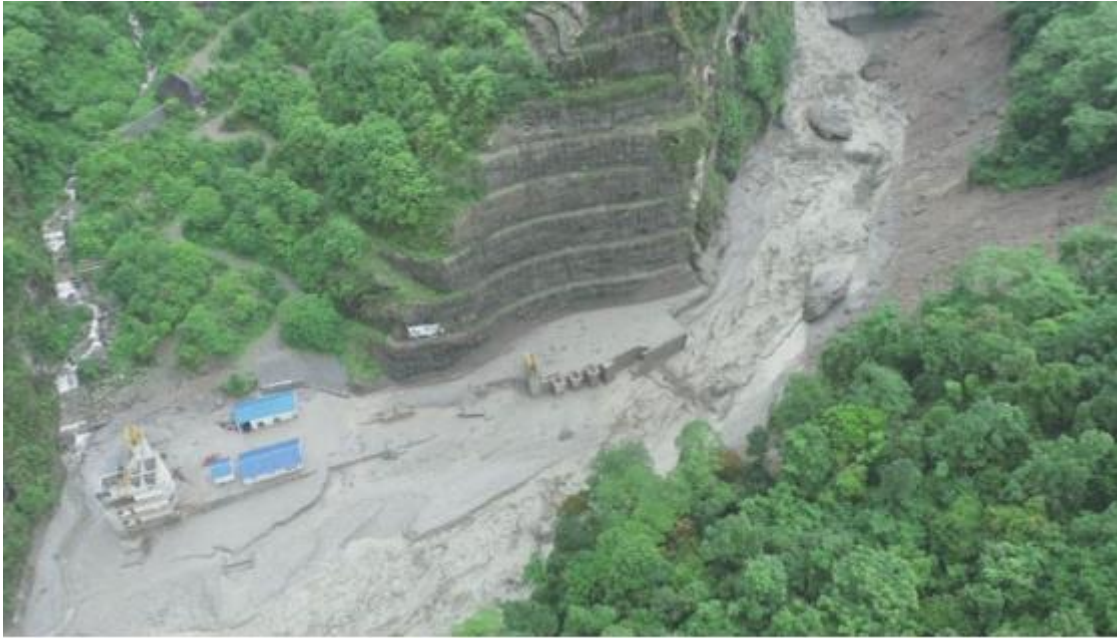
Aerial view of the Melamchi Water Supply Project headworks is covered in mud after Tuesday's flash flood. Eight staff, including Indian and Chinese nationals, are missing.
